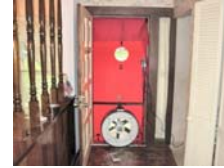
Home energy audits can inform you of leaks and sources of air infiltration.
