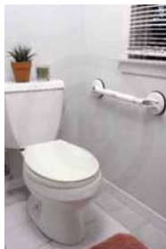
Grab bars next to the toilet and in the tub area assist older adults in the bathroom.
